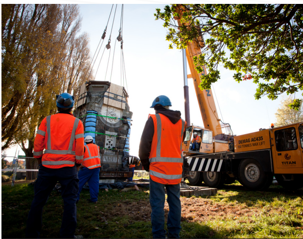
Removal of the top section of Christchurch's historic Edmonds Clock Tower, in preparation for post earthquake repairs and seismic strengthening.
