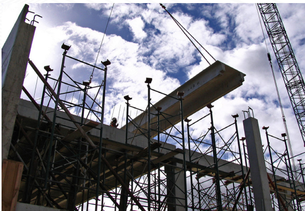
Double tee being placed at the Auckland Airport car park building.
