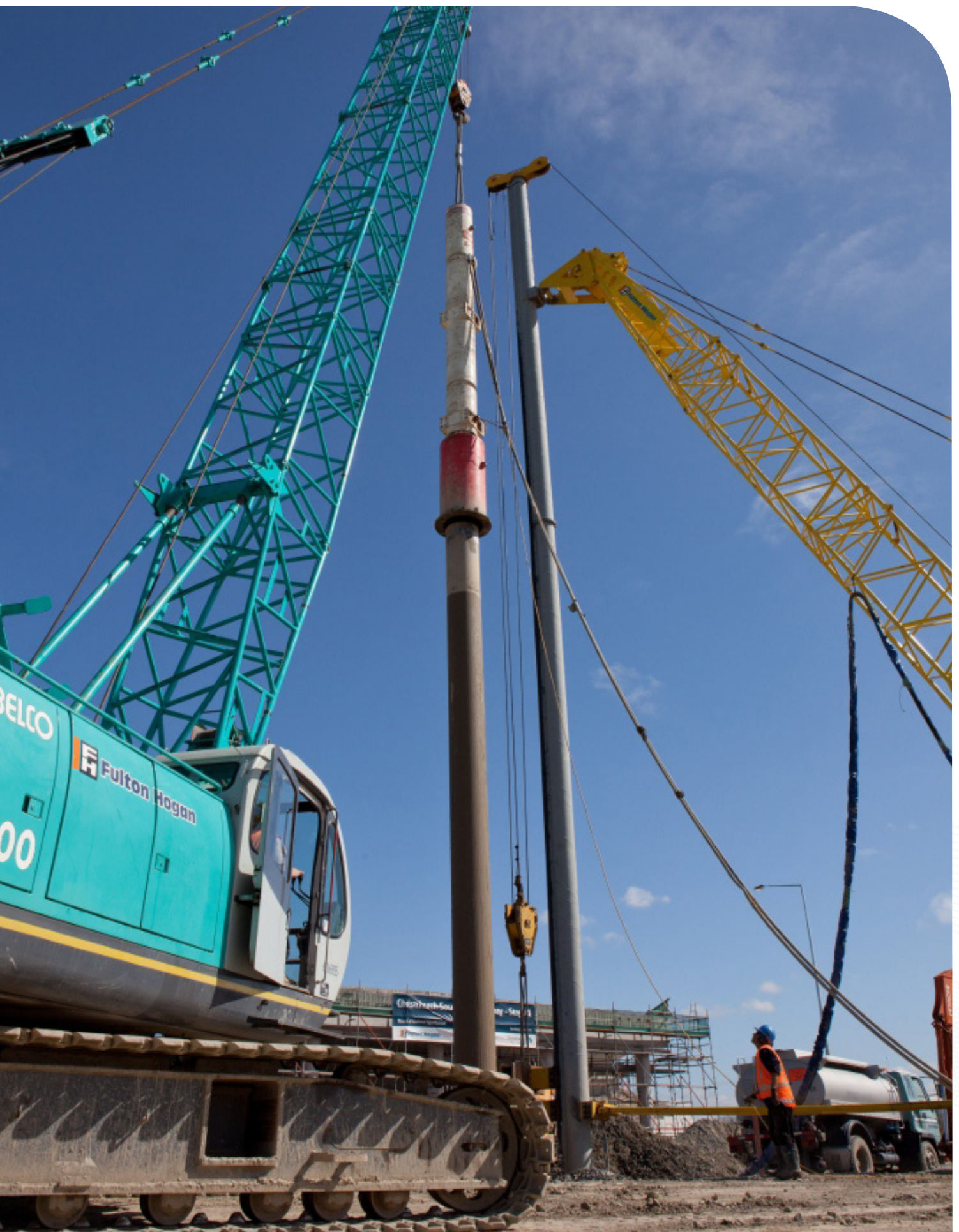
Stone Column ground improvements taking place on the Christchurch Southern Motorway project.
