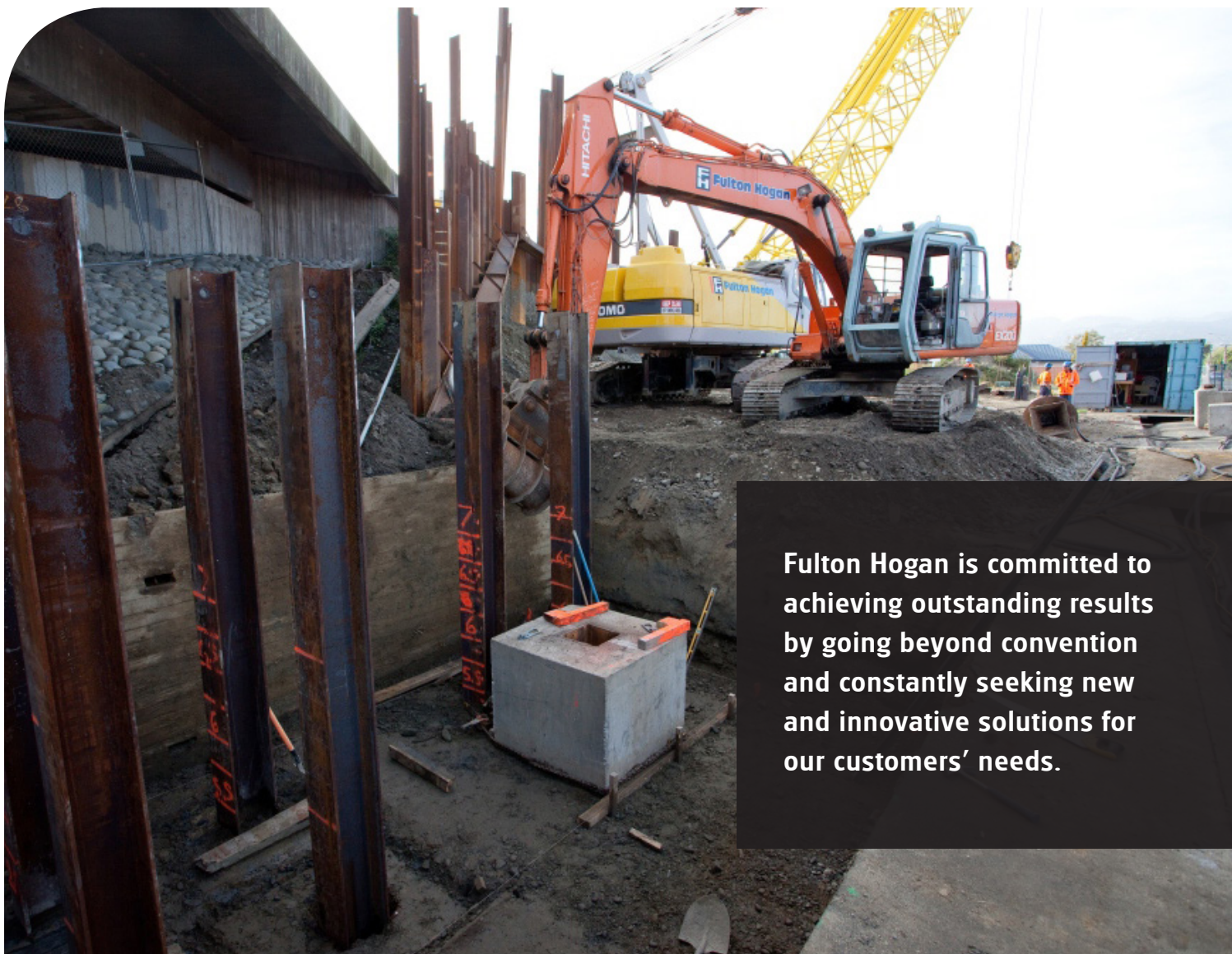
Driven UC Piling at Christchurch Southern Motorway.
