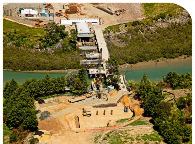
Construction by temporary staging of the Orewa River Bridge in Silverdale, north of Auckland.
