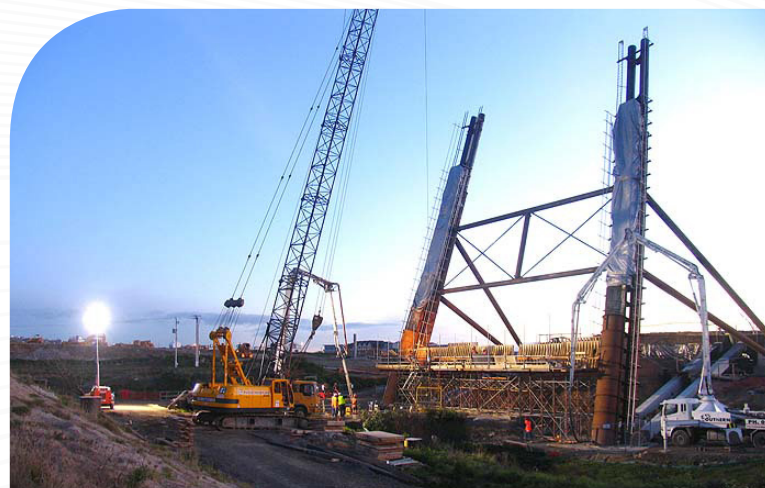
Construction of the cable stay pylon on the Ormiston Road Cable Stay Bridge project in Manukau.
